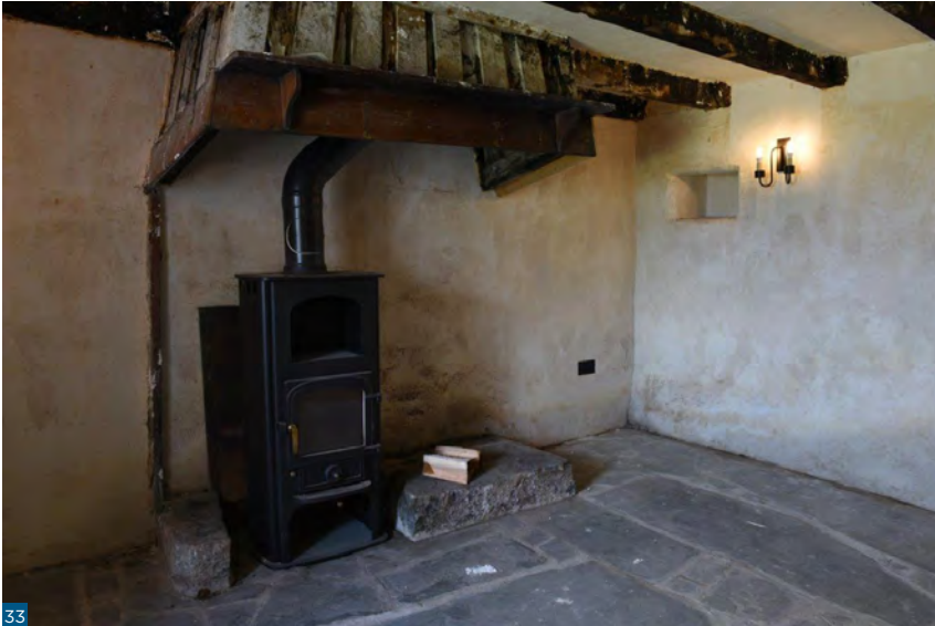
Figure 33: A flagstone floor re-laid on a lime concrete heated slab.
