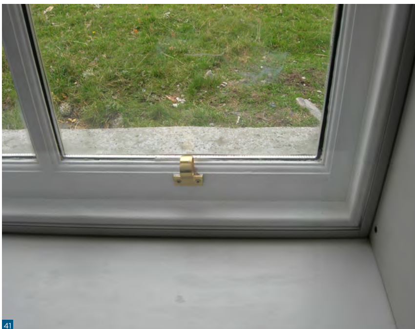
Figure 41: Polycarbonate secondary glazing mounted on a magnetic strip.
