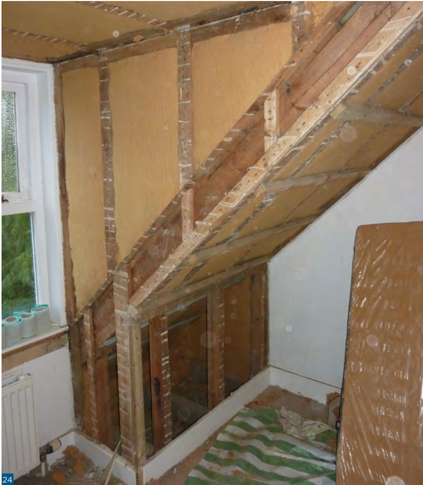
Figure 24: Insulation work to a dormer using wood fibre board.
