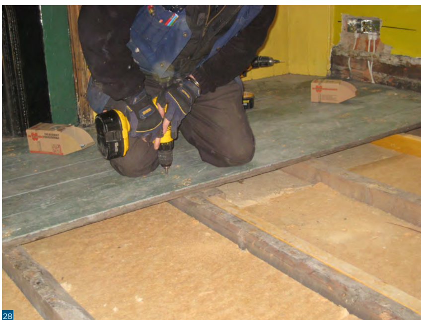
Figure 28: Relaying a timber floor once the insulation is in place.
