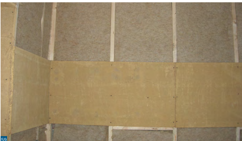
Figure 59: Hemp fibre insulation with clay board.
