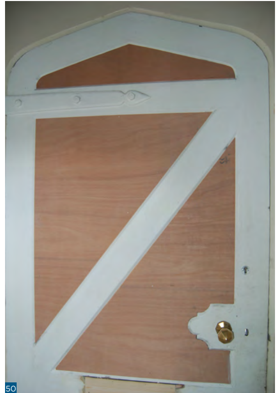
Figure 49: A door in a tenement with the insulation under the new plywood panels prior to painting.
