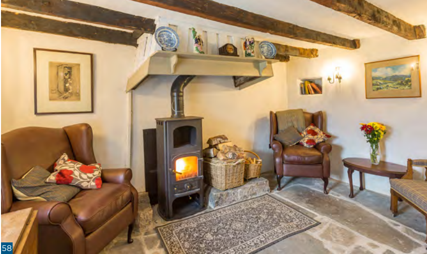
Figure 58: The finished room at Downie's Cottage showing the insulated lime plaster and the re-laid stone flagstones. Image © Callum Innes
