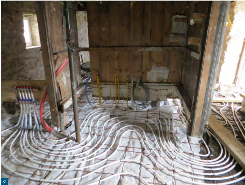
Figure 31: Coils for an underfloor heating system laid on top of a lime concrete floor. The heating is powered by a ground source heat pump. Image © Callum Innes
