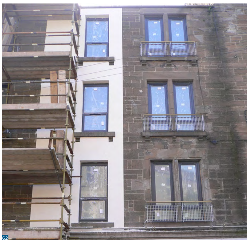
Figure 62: The visual impact of external insulation.
