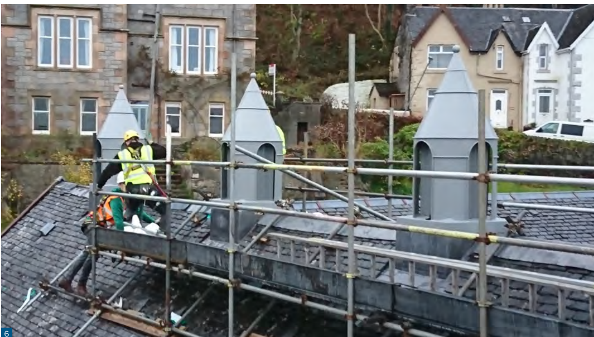
Figure 6: Reinstated ridge level vents at a former school in Oban. Image © Rockfield Centre
