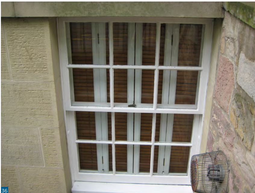
Figure 36: Glazed shutters in use.
