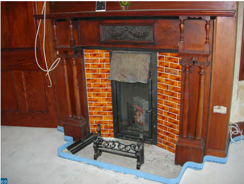
Figure 69: An existing Edwardian cast iron inset retrofitted with a glazed grate for more efficient combustion.
