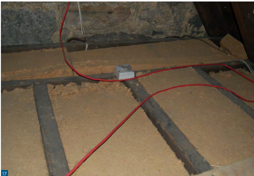
Figure 17: Wood fibre board laid between ceiling joists.
