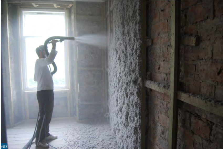
Figure 60: Cellulose insulation being applied damp.
