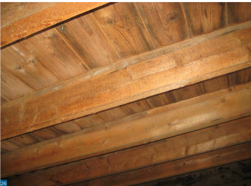
Figure 26: A typical underside of a flat roof.
