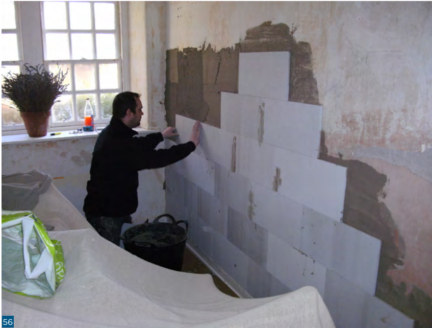
Figure 56: Application of the calcium silicate insulating boards.
