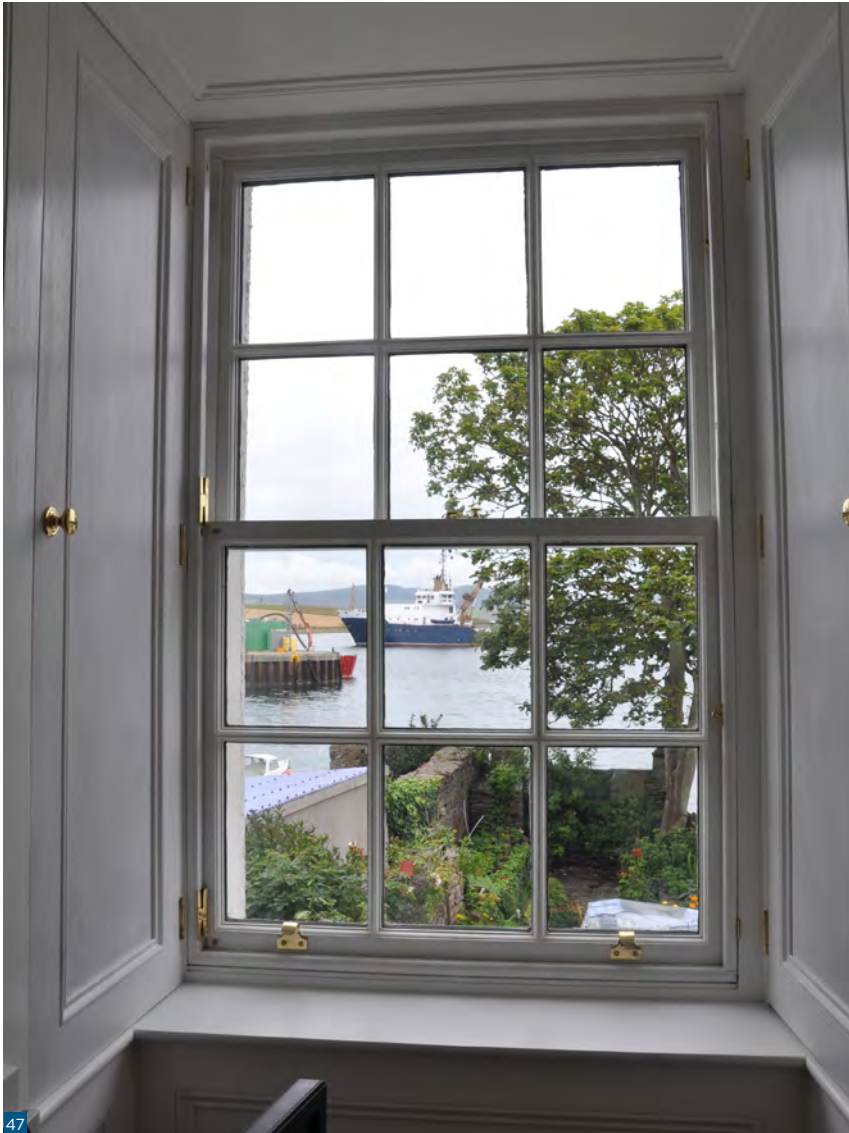
Figure 47: A new sash and case window in a Category B-listed window in Stromness. Note the new working shutters.
