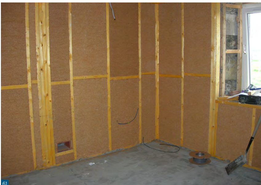
Figure 61: Wood fibre board insulation applied within framing. A U-value of 0.19 was achieved in this example.
