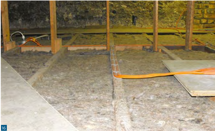
Figure 16: Sheep's wool insulation laid between rafters at Edinburgh Castle. Note the accommodation and fastening of wiring above the insulation.
