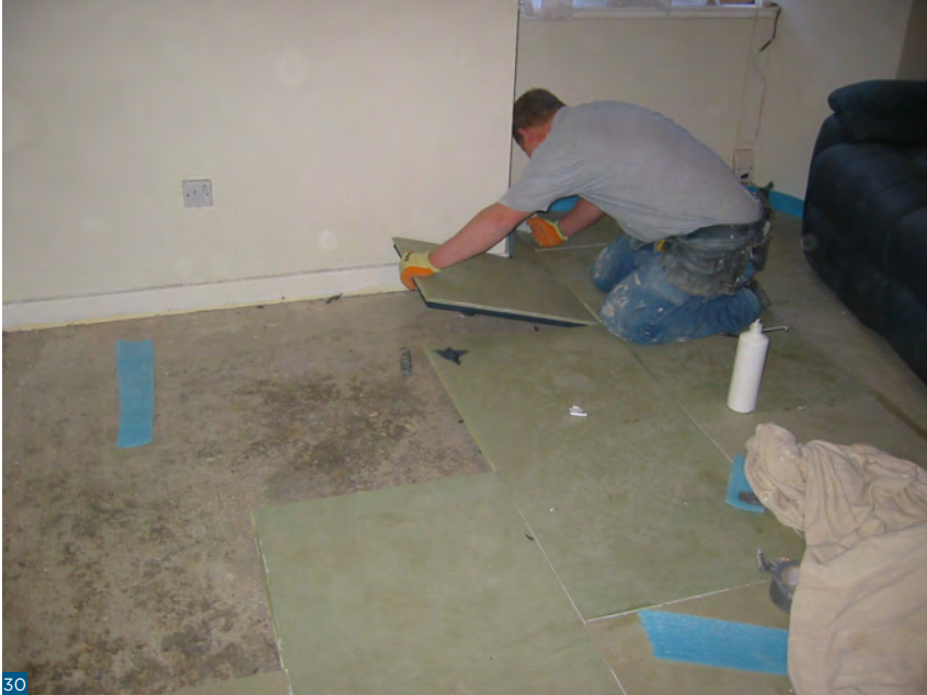
Figure 30: Aerogel board being laid onto a concrete floor. Image © Changeworks
